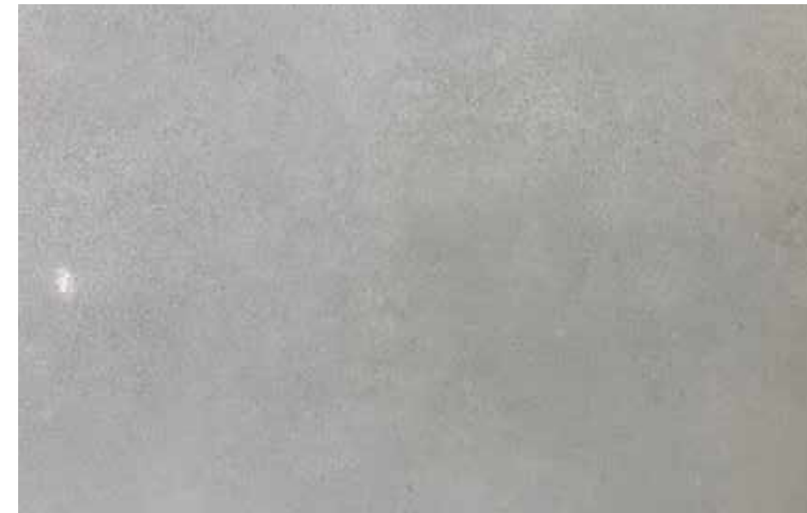
BATHROOM FLOOR AND WALL TILE
